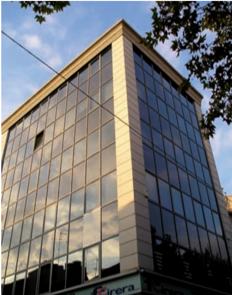
Building housing Bee-Group in Terrassa
