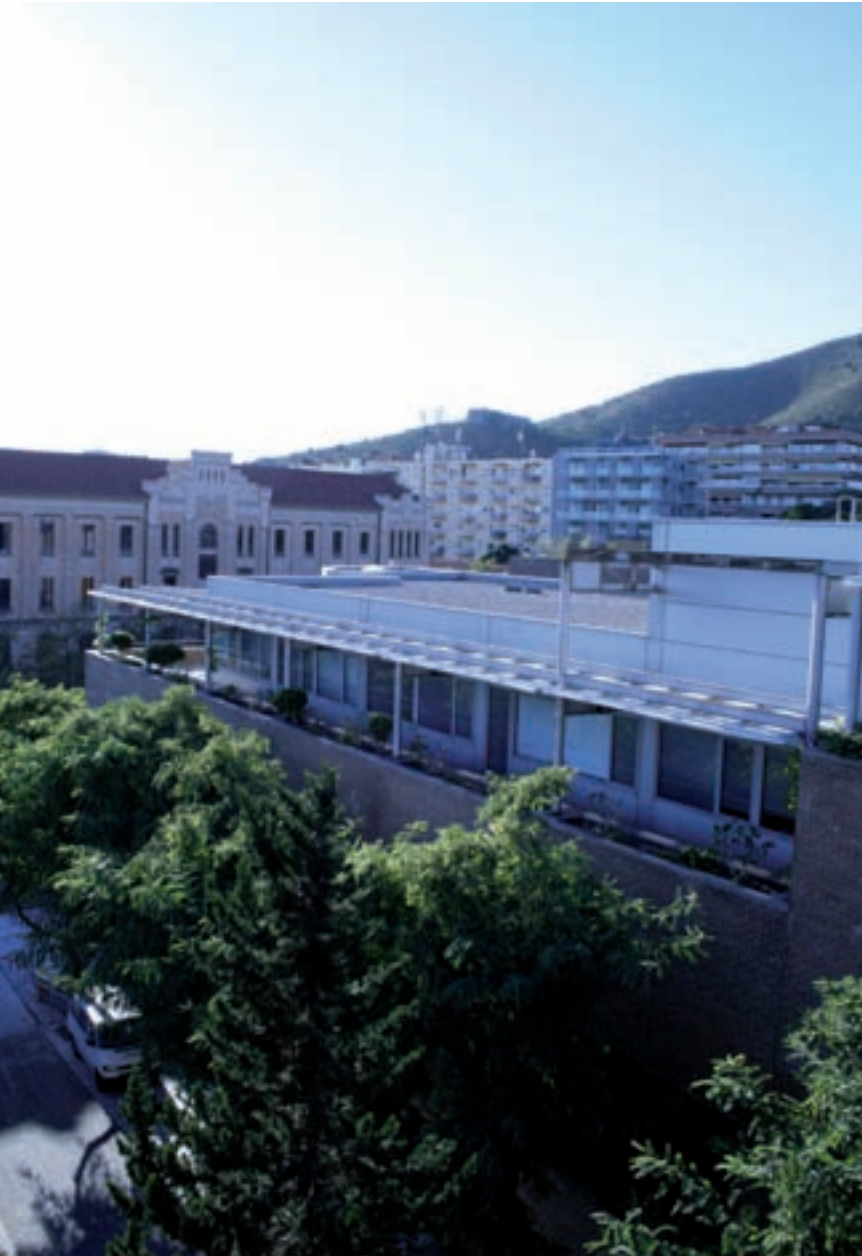
View of CIMNE - Barcelona building
