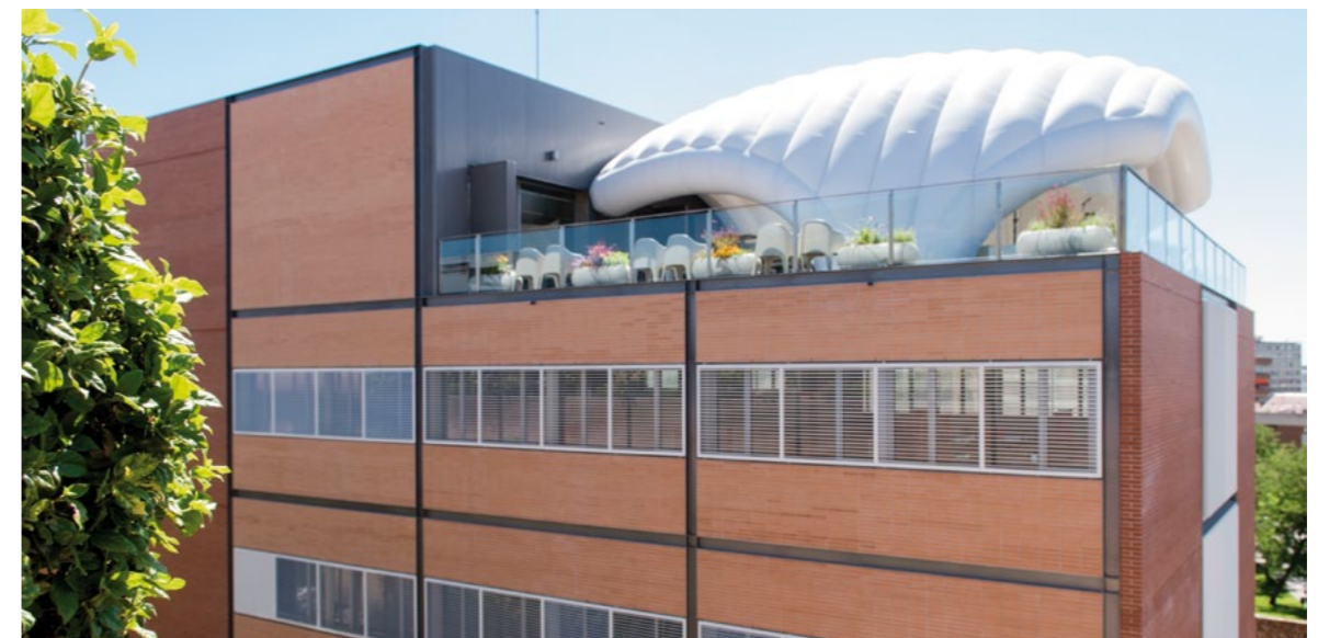
BO Building at Campus Nord UPC Barcelona
