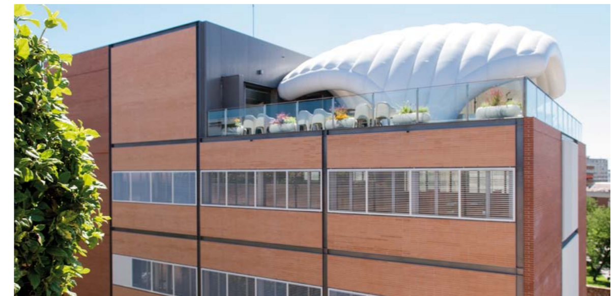
B0 Building at Campus Nord UPC Barcelona
