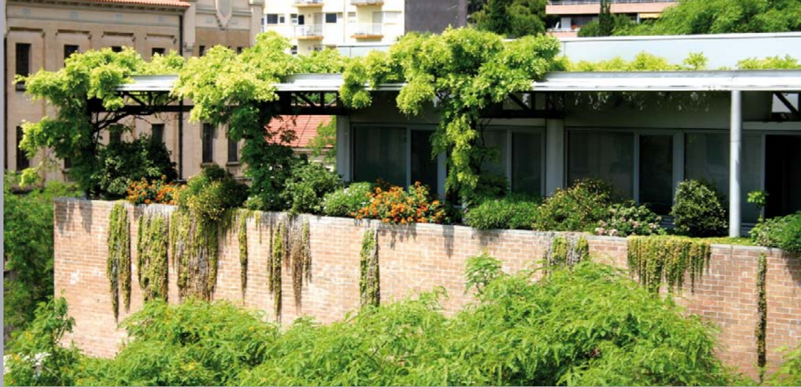
C1 Building at Campus Nord UPC Barcelona
