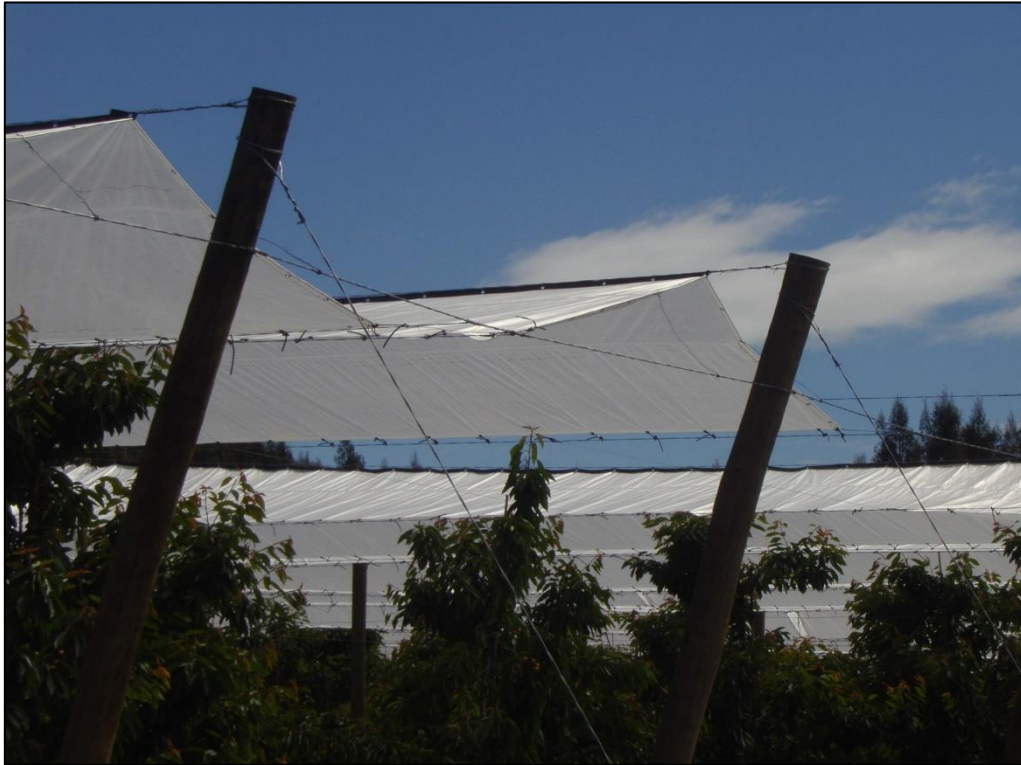
Figure 1: Installed Tents in Chile
