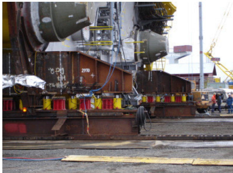
Fig 4.7 Skidding by uniform loading using hydraulic cylinders
