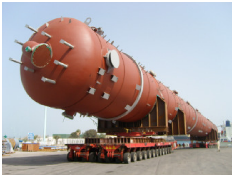
Fig 4.5 Roll-off operation of a heavy-lift on SPMT
