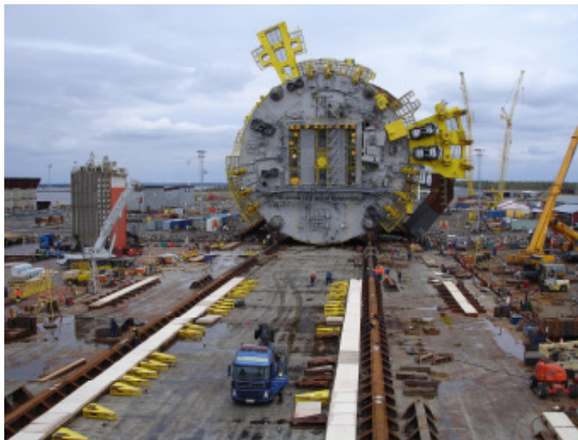
Fig 4.6 Skidding of a SPAR
